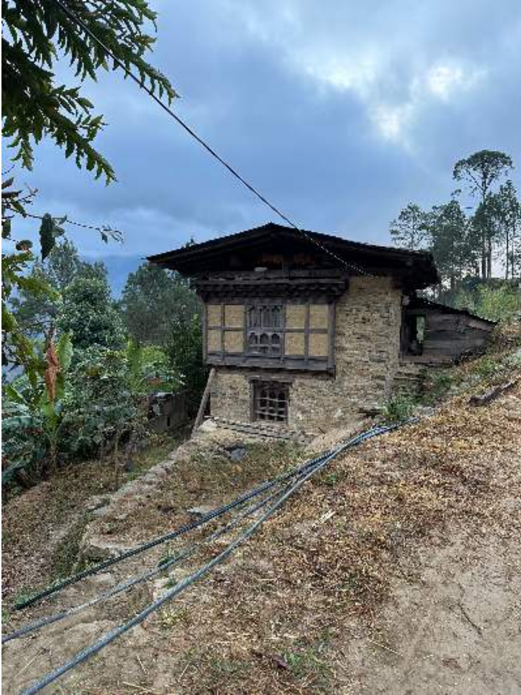
Monpa house with power lines above and water lines along the ground
